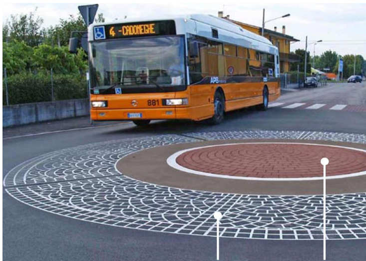
Image 2: The roundabouts can help in maintaining constant traffic flows at lower speed. Source: General Spatial Plan of Glyfada, PRISMA, 2016
