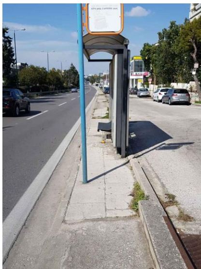
Image 10: Bus stop on Vouliagmenis Highway. There's no adequate pavement or acces ramps. Very small waiting area and at a very short distance from the high speed traffic.
