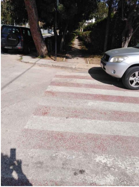
Image 8: Crossing on D. Gounari street (tennis courts) without an accessibility ramp and high speed traffic
